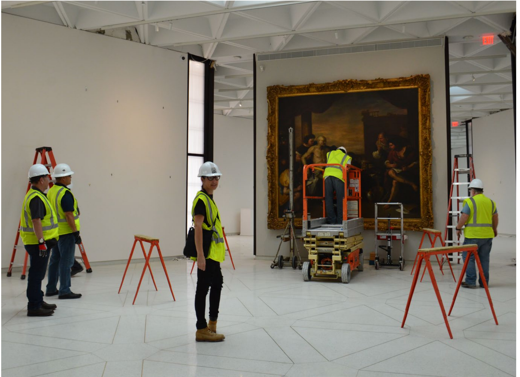
Earthquake emergency recovery
